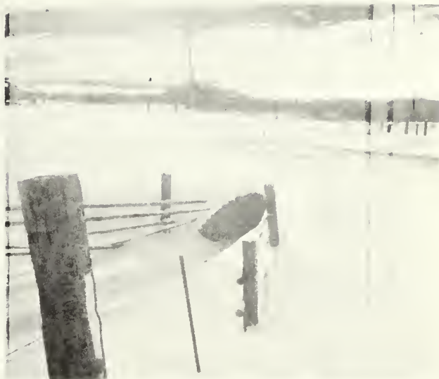
SOUTH ENTRANCE; Snow is about 2' deep, drifting to 6' adjacent to entrance.
